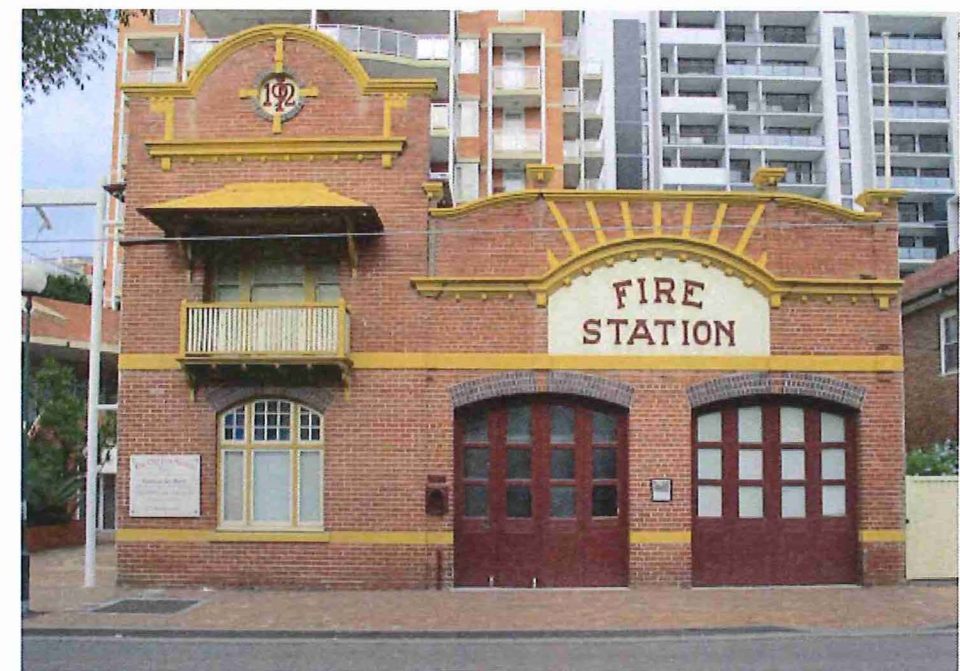
SITE PHOTO 2 - HERITAGE FIRE STATION
